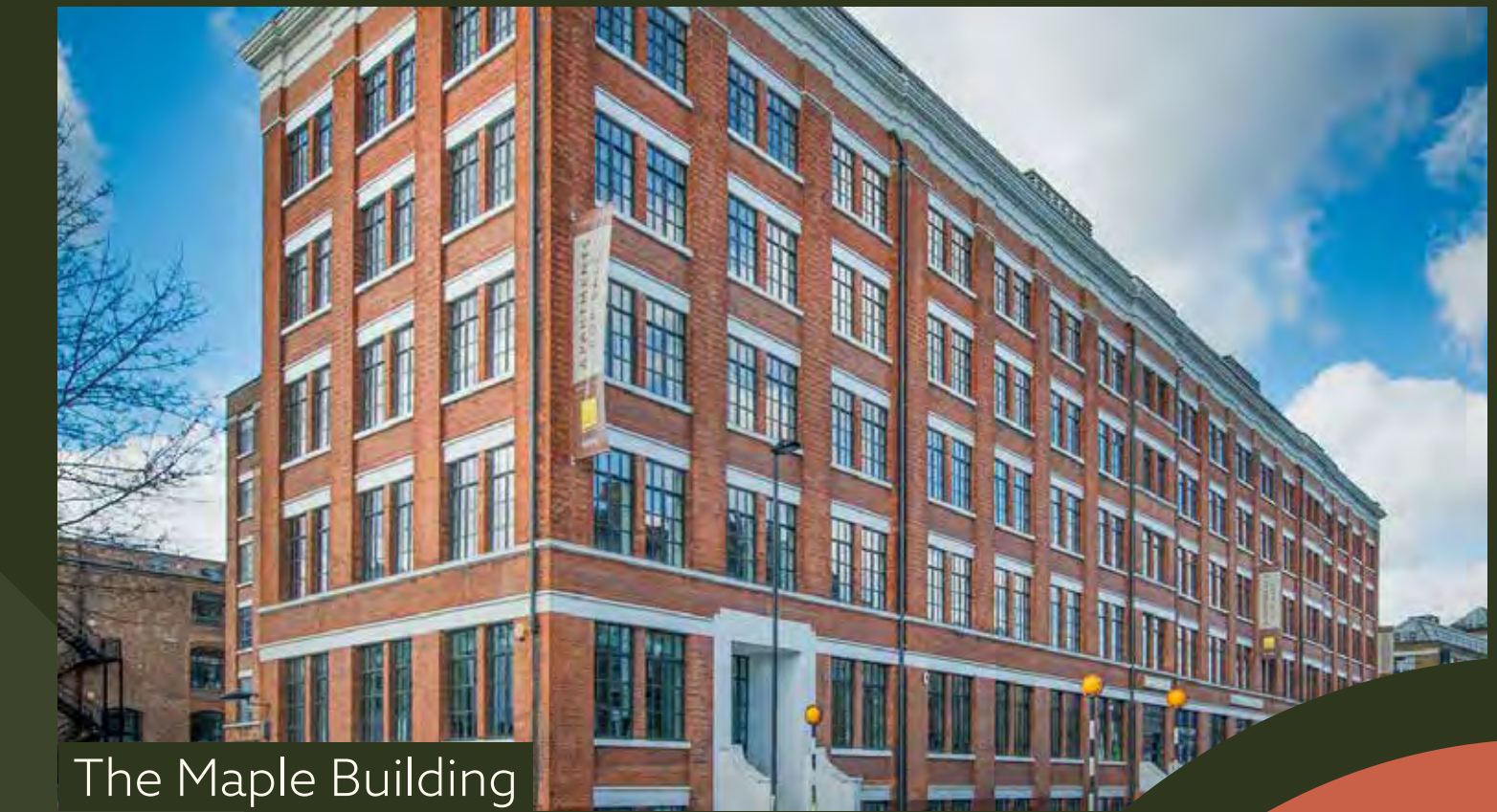
The Maple Building
